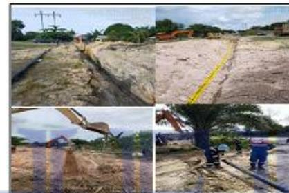
Segmen 5 : Aktifitas Trenching, Lowering, Pengukuran Top of pipe, di KP 7+000 - KP 7+500
