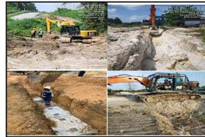
Segmen 5 : Aktifitas Clearing di KP 5+700, Instal concrete slab 8+900, Trenching, Backfill di KP 7+600
